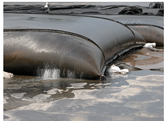
Geotube Dewatering
