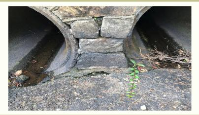
This is a picture of the western spillway taken in the summer of 2023. You can see that the mortar between the stonework has begun to erode and is in need of being repointed. More importantly, while the spillway is dry, water continues to drain beneath the infrastructure of the spillway itself. This is a sample of the maintenance issues of the dam that this project will rectify.
