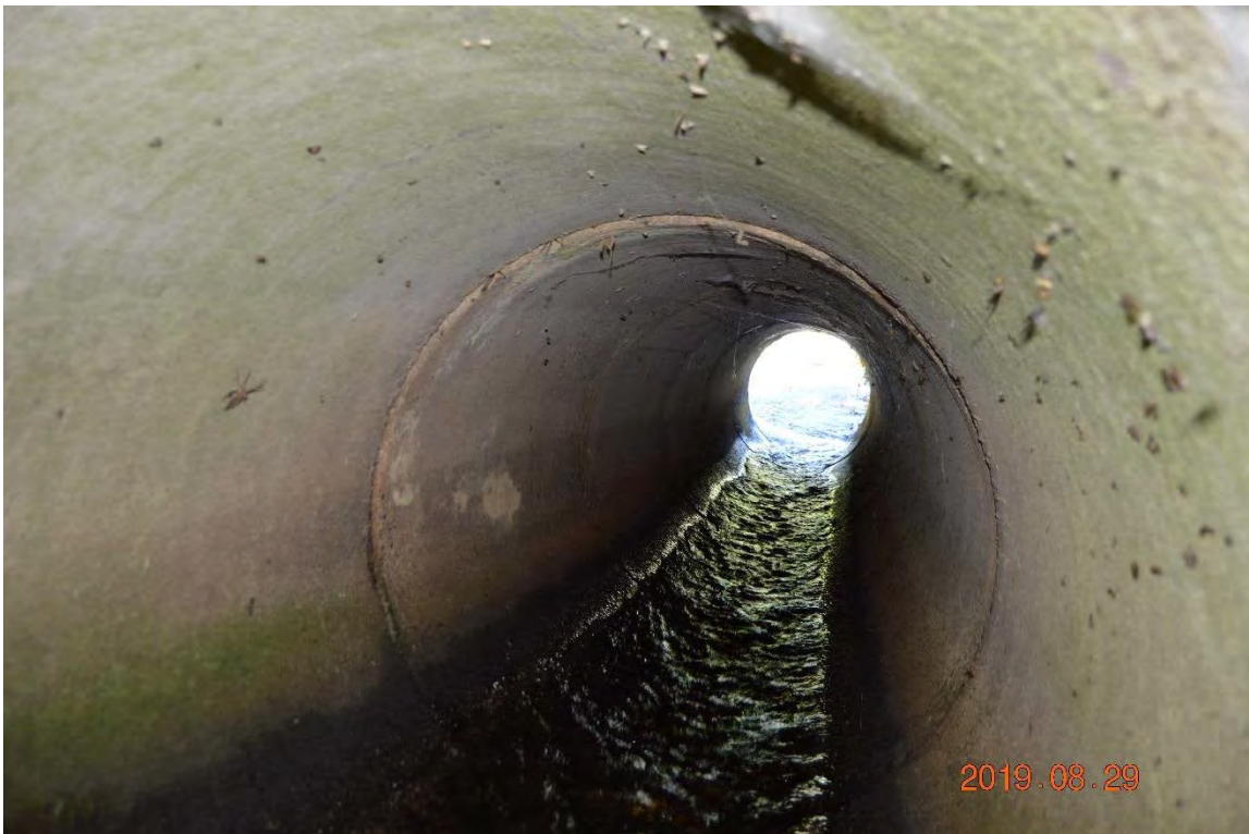
Photo 19d – The interior of the left of the twin right side outlet pipes, in good condition and representative of both pipes.
