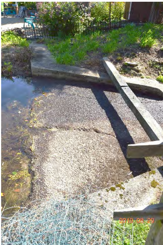
Photo 4b – The short upstream embankment section to the left of the left side spillway. Care must be taken to establish a good grass cover here.
