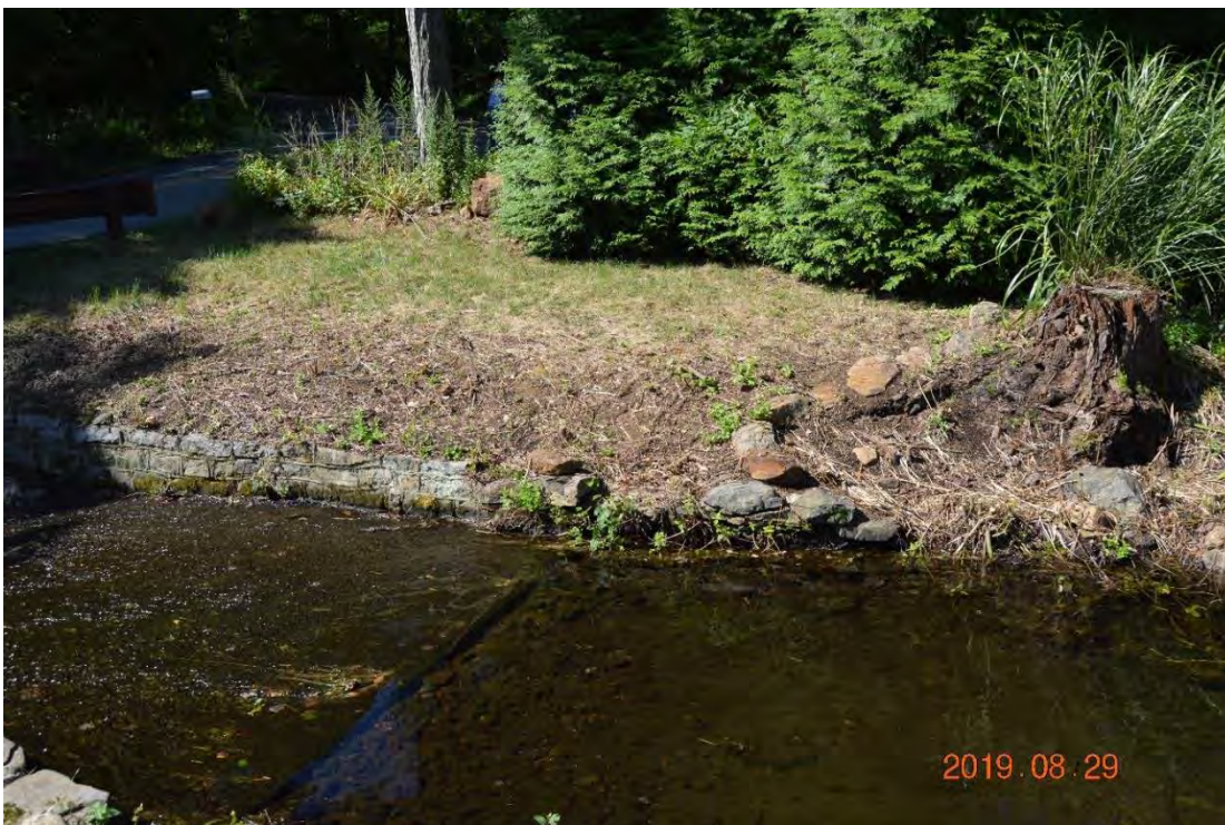
Photo 21b – The embankment along the right side of the right discharge channel. This area was recently cleared of brush and vegetative growth, and should have a grass cover established and maintained. The tree stump (from previous clearing) must be monitored and any depression resulting therefrom filled in as required if subsidence should occur. In the event of reconstruction of the training wall area, the stump and roots should be removed at the same time. The training walls in this area have deficiencies that require improvements and repairs.
