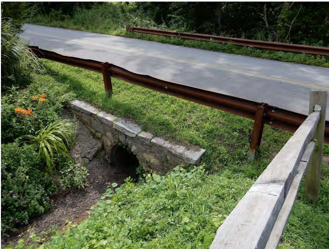
Photo 19b – The upstream end of the left side outlet pipe and headwall.
