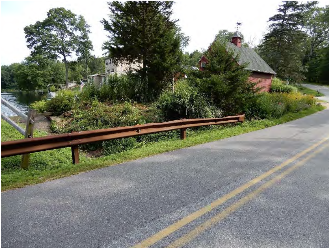
Photo 8b – The left side downstream embankment face (to the left of the left side spillway), prior to the removal of brush and vegetation.
