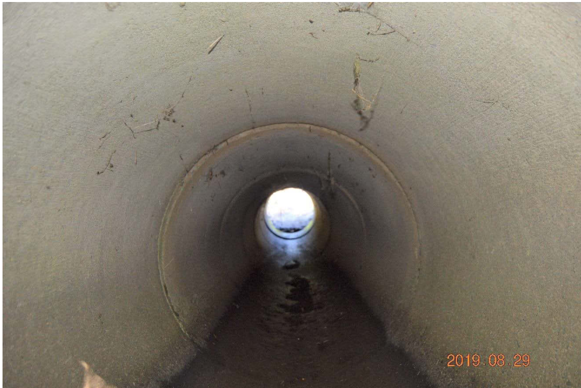
Photo 19g – The interior of the left side outlet pipe, in similarly good condition to the two right side pipes.
