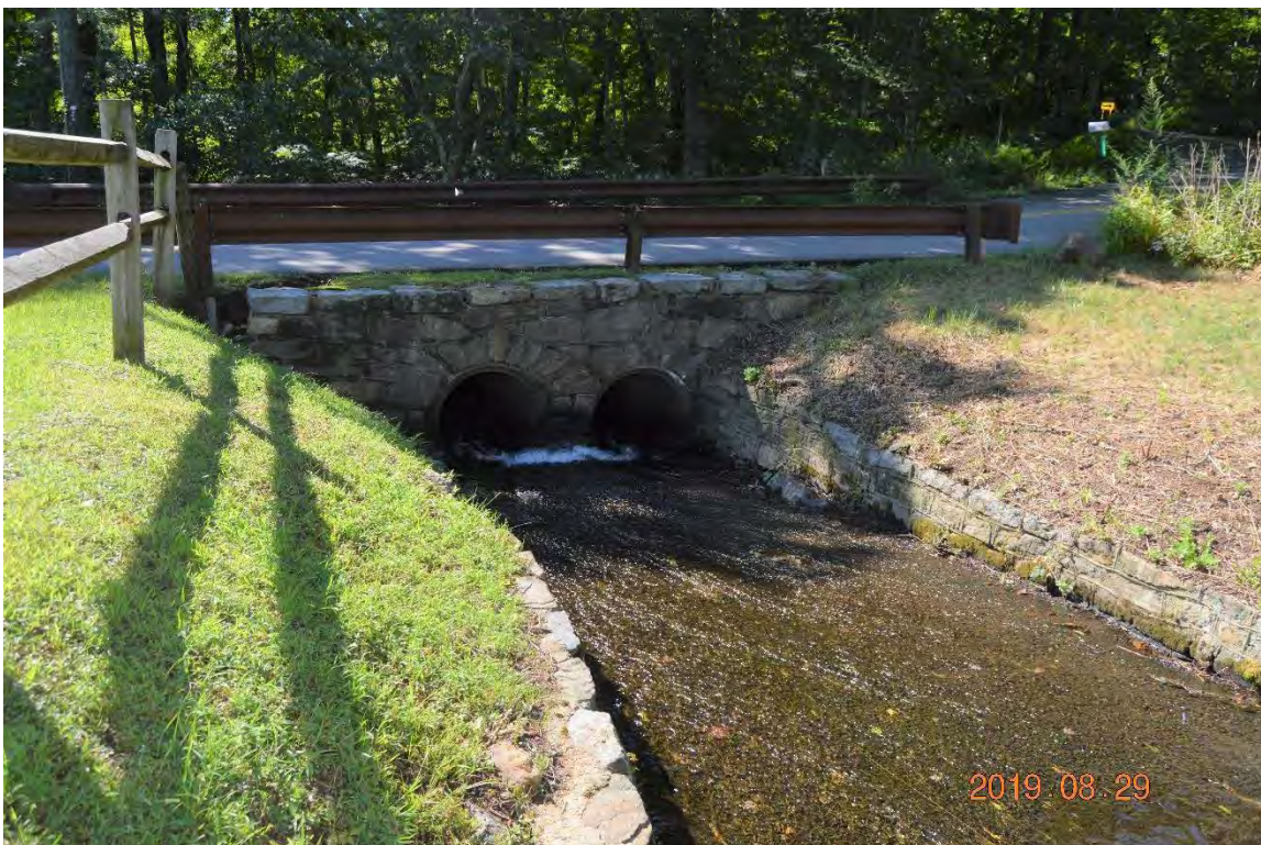
Photo 15c – An overview of the right side discharge channel as seen from the upstream side, following the removal of brush from the right side embankment. Note the two barrel culvert at the downstream end of the channel.
