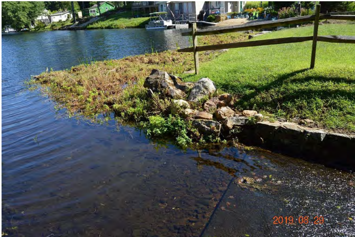
Photo 3d – The junction of the upstream embankment with the right side spillway.
