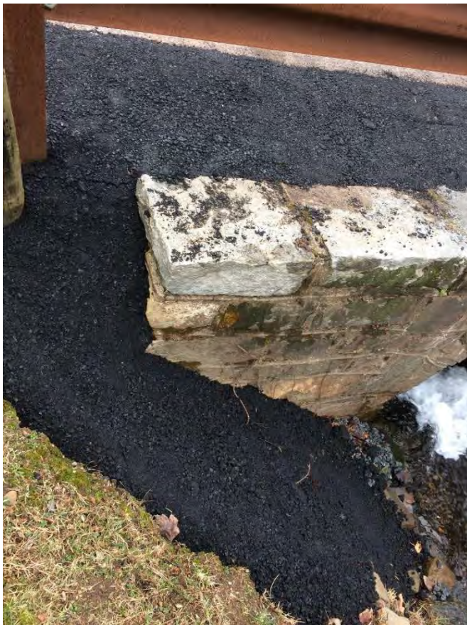
Photo 21c – An area of washed out soil, caused by runoff from Haywardville Road, running around the right side discharge culvert endwall at the time of inspection. This area was subsequently repaired (see below).
