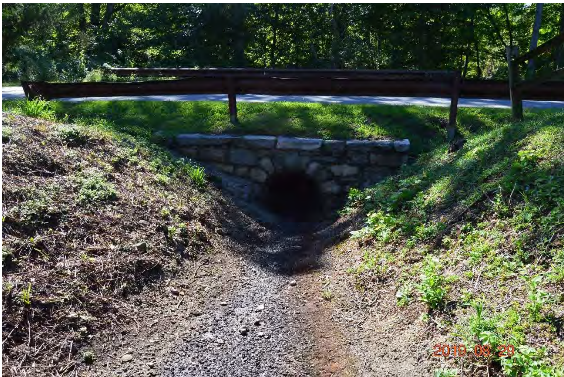
Photo 21f – The lower portion of the left discharge channel. Side slope areas where brush growth was recently cut must be kept cleared with the reestablishment of a grass cover to prevent erosion during high flow situations. (See Section XII for additional long term recommendations.)
