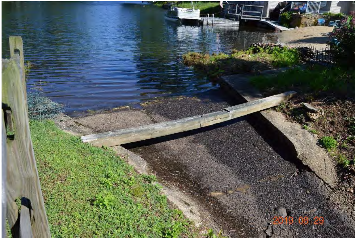
Photo 13a – The left side spillway weir.
