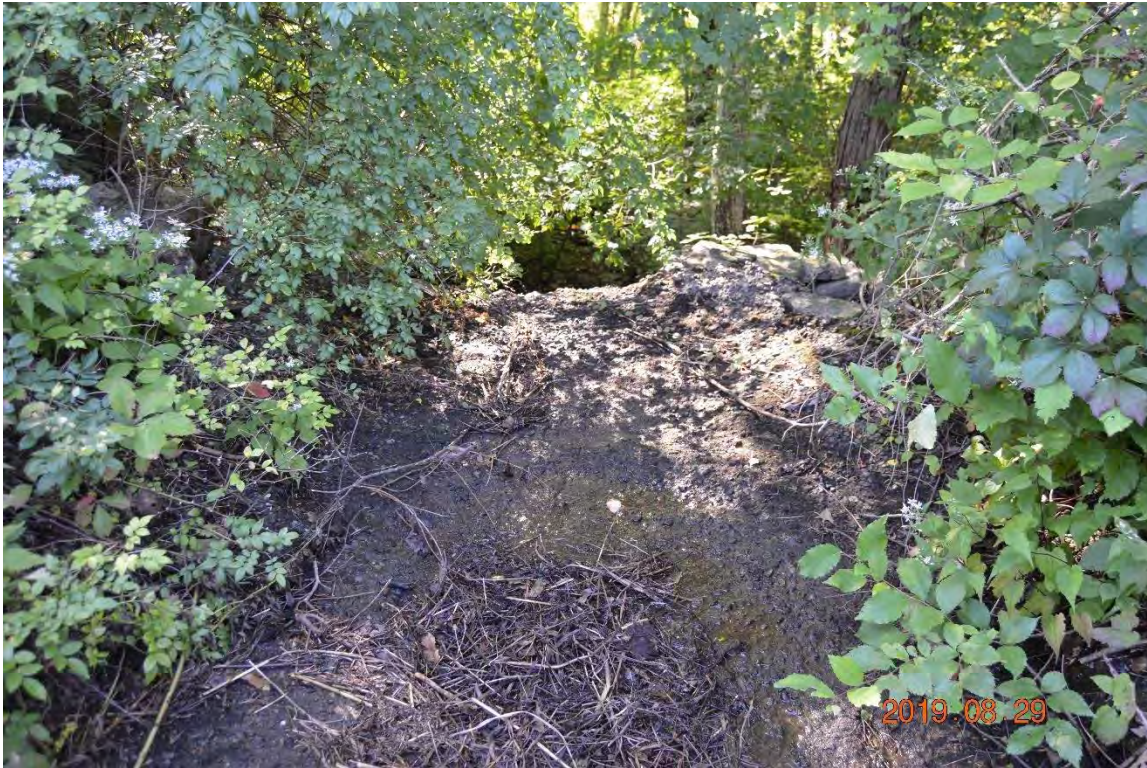
Photo 15f – The left side discharge channel stretching away beyond the apron at the base of the outlet pipe. At the upper center of the photo is a retaining wall from the old mill site, with a drop to the base channel of about 8 – 9 feet.
