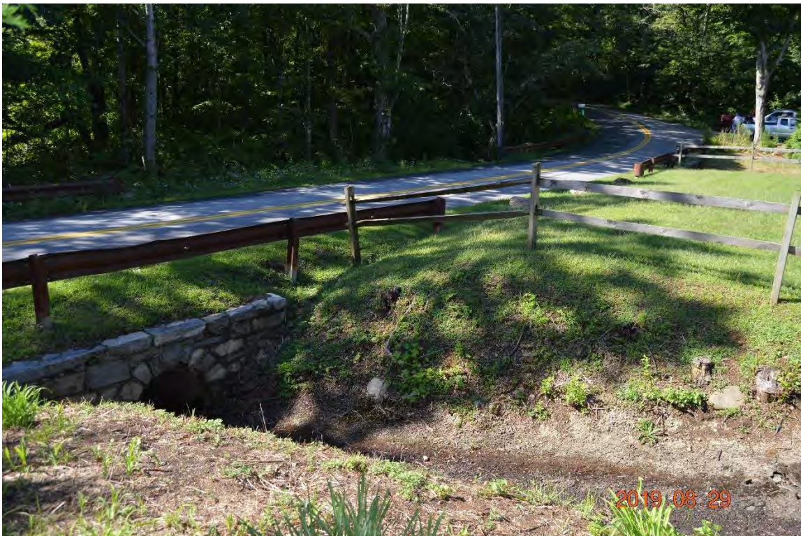
Photo 8c – Another view of the downstream embankment taken from the left side, with the transition to the left side discharge channel in the foreground and with tall vegetation removed.
