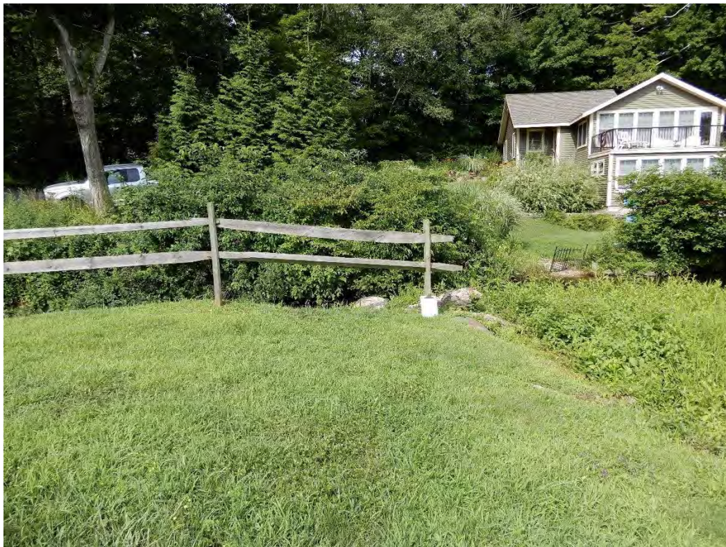
Photo 3a – The right upstream embankment face, prior to removal of vegetation completed between the two inspection dates.
