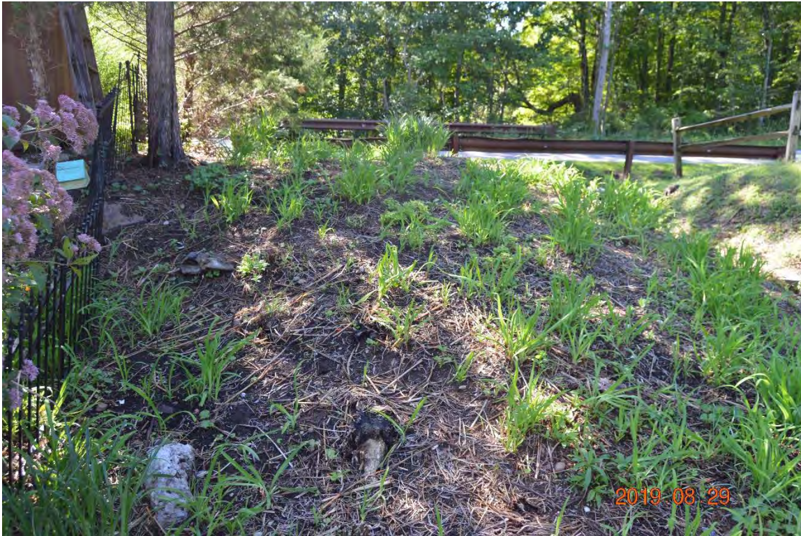
Photo 4b – The short upstream embankment section to the left of the left side spillway. Care must be taken to establish a good grass cover here.
