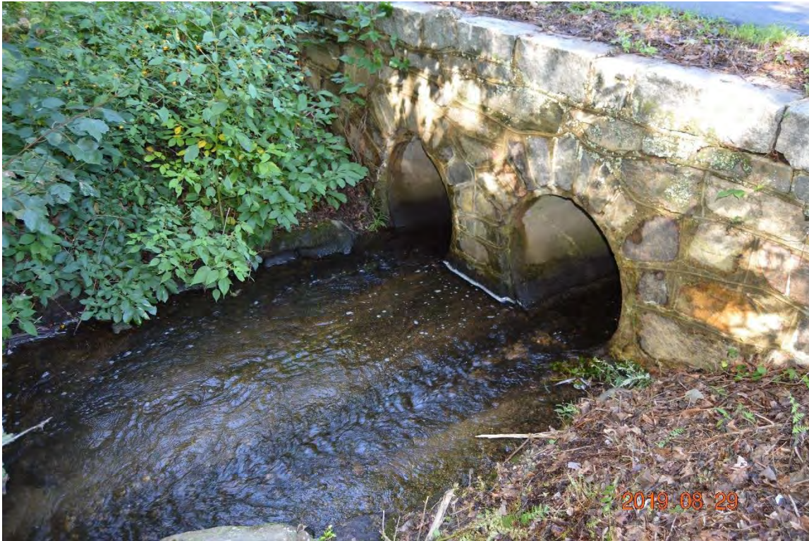
Photo 19c – The downstream end of the right side outlet pipes. The endwall is in good condition.
