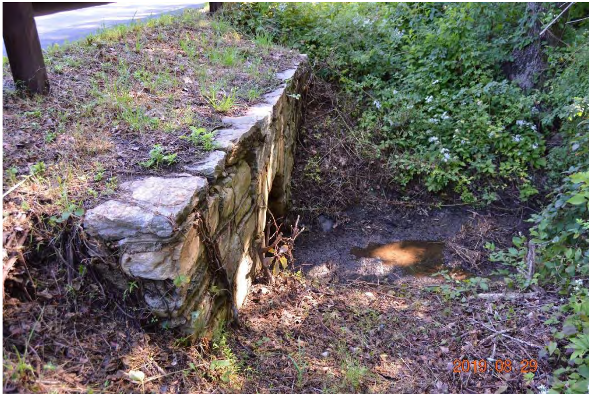
Photo 19e – The downstream end of the left side outlet pipe. This endwall is also in good condition.
