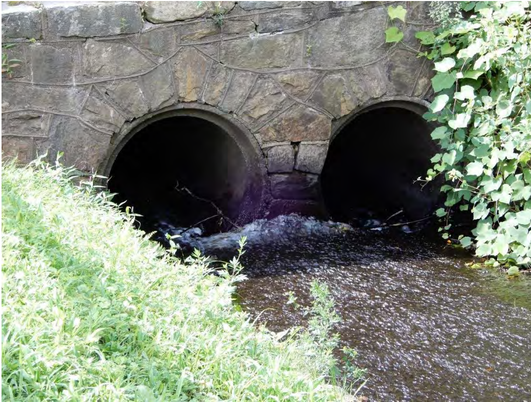
Photo 19a – The upstream end of the right side outlet pipes and headwall.
