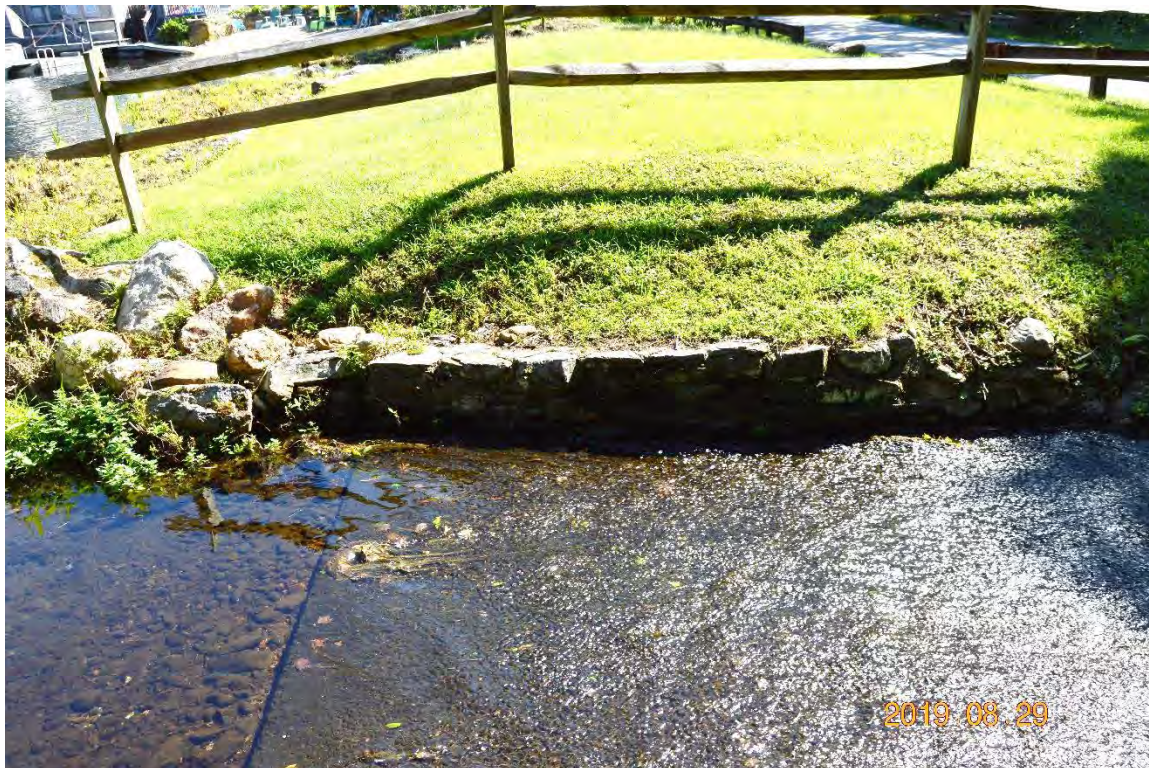
Photo 13b – The right side spillway weir.
