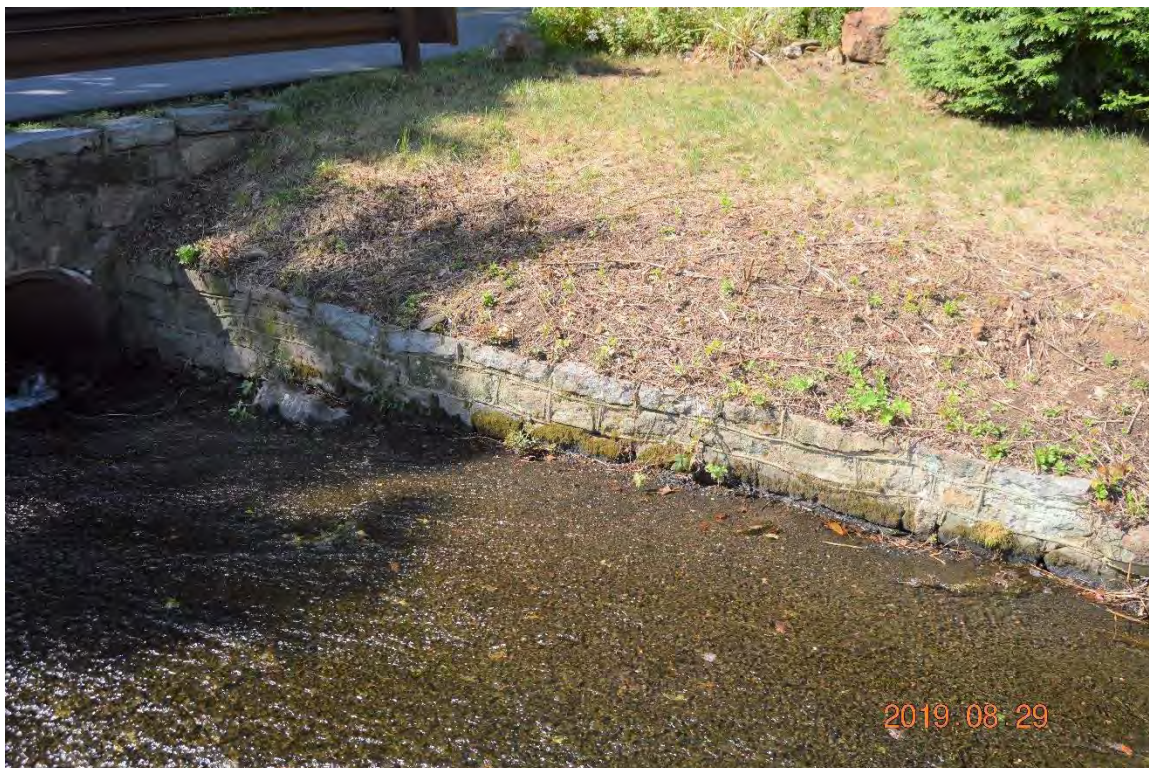
Photo 11a – The right side channel training wall along the discharge channel emanating from the right side spillway.
